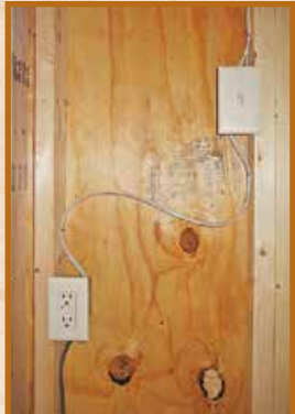
Wired for Electricity
